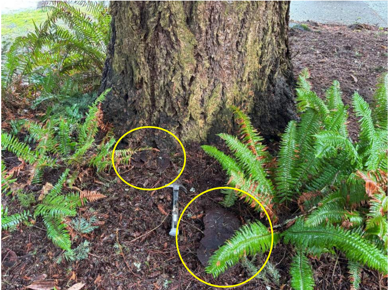
Photograph 4. P. schweinitzii fruiting bodies, circled above, observed south/southwest of the base of tree 401. If the tree is retained, I recommend an advanced assessment by microresistance drill to test for sound wood.
